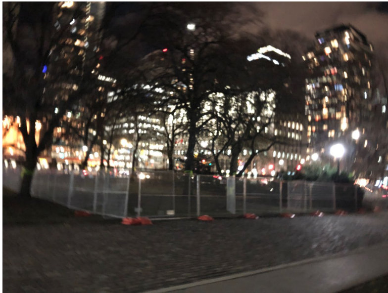
Friday night, December 9, 2022 Fence erected by Metrolinx
